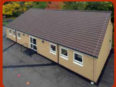
Characterised by their high, bold roll profile and manufactured with a choice of through-coloured or granular finishes in nine different colours, the Regent tile offers flexibility and compatibility to suit all roof types. Due to its low pitch capability, Regent can be specified for roofing designs with a pitch as low as 12.5°
