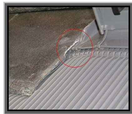
“ Notch “ at aluminium fold
