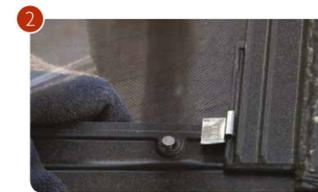
(i) Position the Verge Clip to ensure overhang of 38-50mm.
