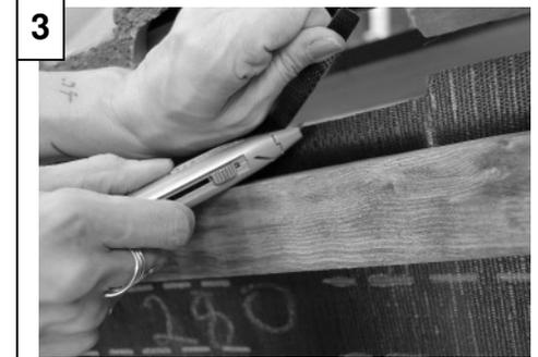
Cut the underlay along the chalk lines with a sharp knife. If sarking is also present, a section of this must also be removed to provide a clear 280 x 50 mm path into the roof space.
