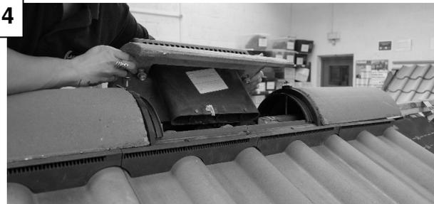
Place the Terminal through the hole in the underlay (and rigid sarking). For Dry & DryVent Ridge, place Profile Filler Unit below the Terminal and secure with the drive screw and clamping plate provided in the pack. For mortar bedded ridge, continuously edge bed and solidly bed ends of the Terminal.
