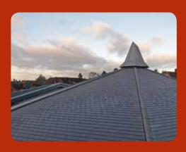
Redland Cambrian Slates embody the beauty and character of natural slate, manufactured in Wales with over 60% recycled Welsh slate. Interlocking, they are made to meet the latest performance requirements and, whilst light in weight, Cambrian's unique three-point fixing makes them suitable for even the most exposed sites.
