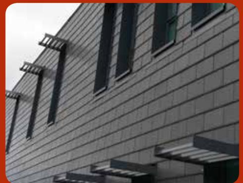
Redland Cambrian Slates embody the beauty and character of natural slate. Manufactured in Wales from 60% recycled Welsh slate with a thin leading edge. Interlocking, they are made to meet the latest performance requirements and, whilst light in weight, Cambrian's unique three-point fixing makes them suitable for even the most exposed sites.
