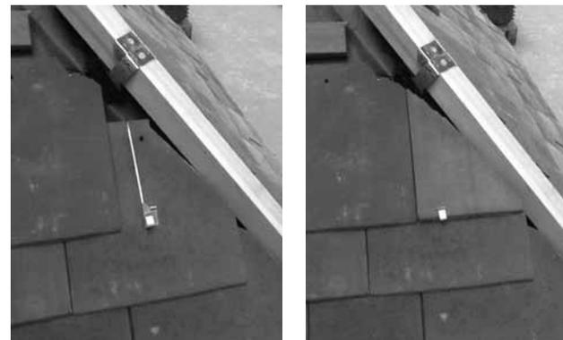
Bend the end of the Tail Clip over the tile on the course below and slot the cut piece into the clip.
