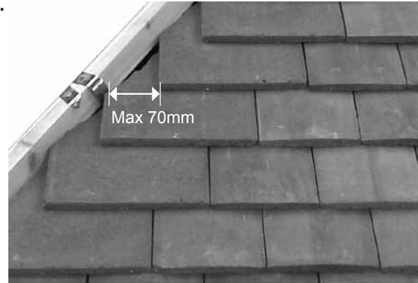
All perimeter tiles should be mechanically fixed with either nails or clips.
