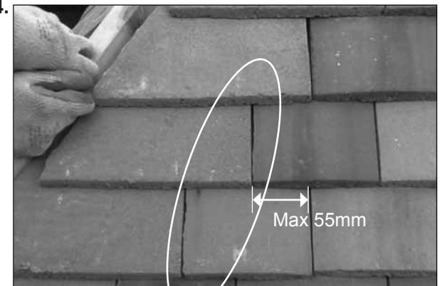
If the maximum 70mm gap cannot be achieved with a Plain Tile-and-a-half or a Plain Tile, then cut the tiles back into the course to reposition the end tile and reduce the gap.
