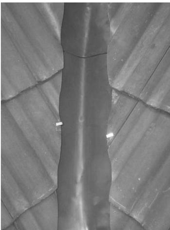
Complete the installation of the valley as shown in diagram in Section 1.1. At the top of the valley a Rapid Flashing saddle will be required. At the eaves, ensure the Rapid Flashing welt is turned out and splayed into the eaves gutter.
