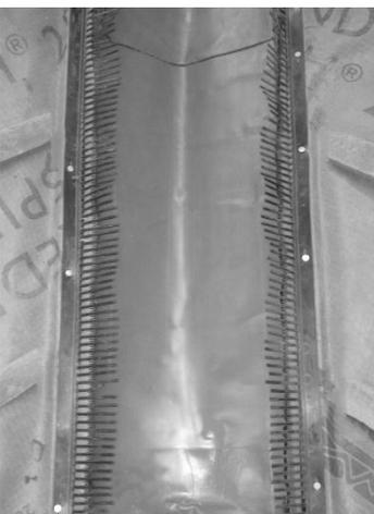
Continue fixing and laying the Rapid Flashing lining up the length of the valley with an 150 mm overlap between lining pieces. Ensure a roller is used with each piece to dress the lining into the valley support board, and to ensure that each lining piece bonds to the piece below. For each piece also ensure the integrity of the glue seal between the Rapid Flashing and the underlay on top of the support batten on either side of the valley is maintained.
