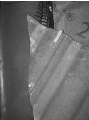
The recommended combination of clips is to use C-clips both at the head and tail of the cut tile at the coverlock/interlock junction with the tile adjacent, and a Kro-clip on the free cut edge of the tile overhanging into the valley. Ensure the C-clips fit tightly to the cut tile. This provides a very secure three-point fixing for the cut tile as shown.
